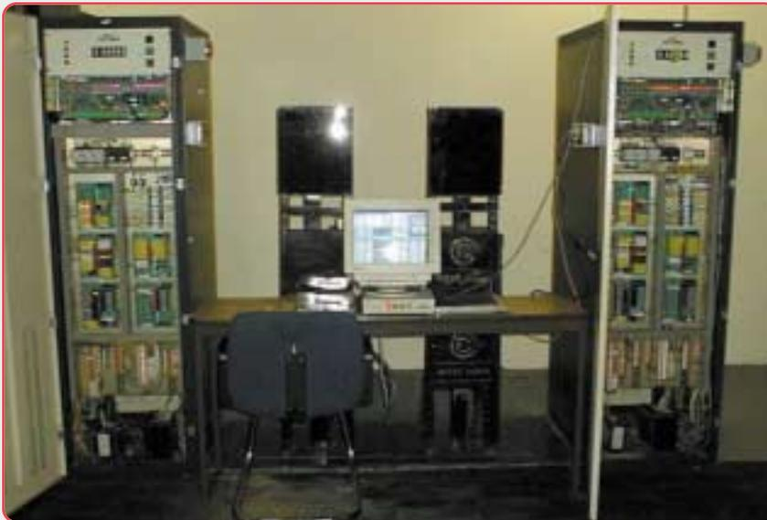
Elevator machine room showing typical installation of SWIFT controller
